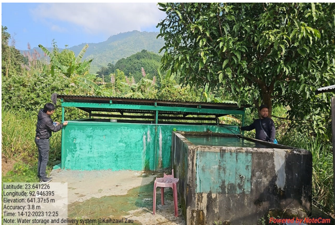
Monitoring of Water Storage & Delivery System, Saitual District
