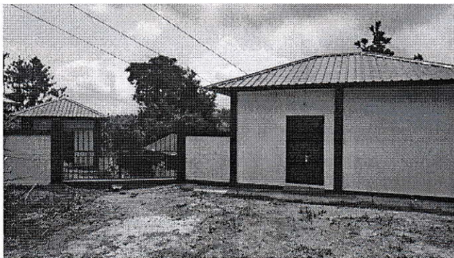
BSS entrance with Changing room
