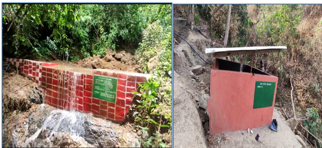
Pic showing Checkdam and Water Storage Tanky
