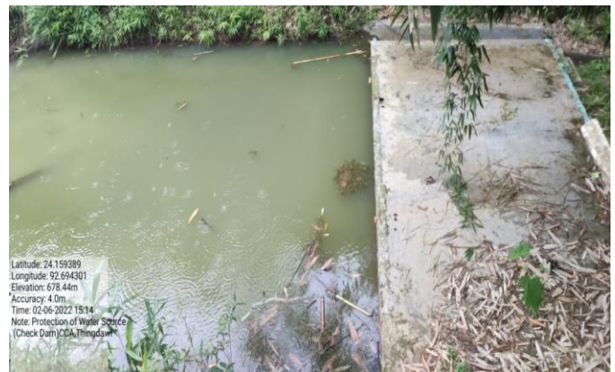
PICTURE2: AFTER CONSTRUCTION
