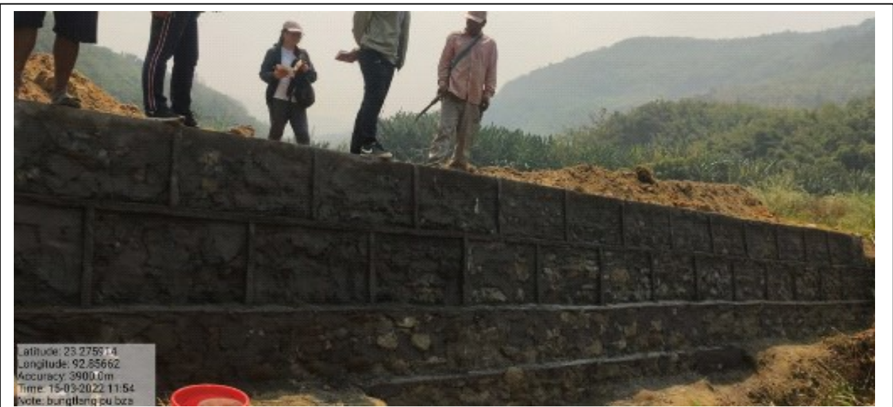
Before and After construction of Gabion Box at Chekawn ( C.Vanlalhruaia)
