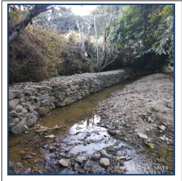
Stream line straightening to reduce soil erosion at WRC area, Chekawn
