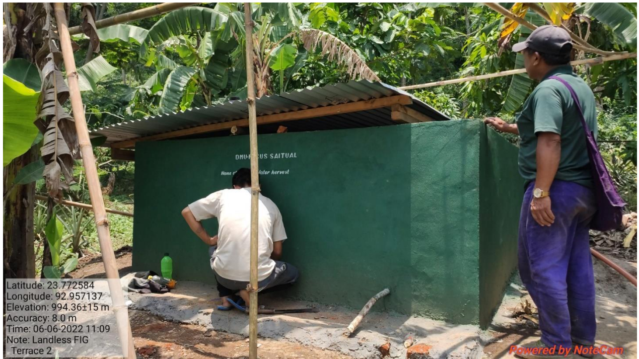
FIG 3: Depiction of few completed work
